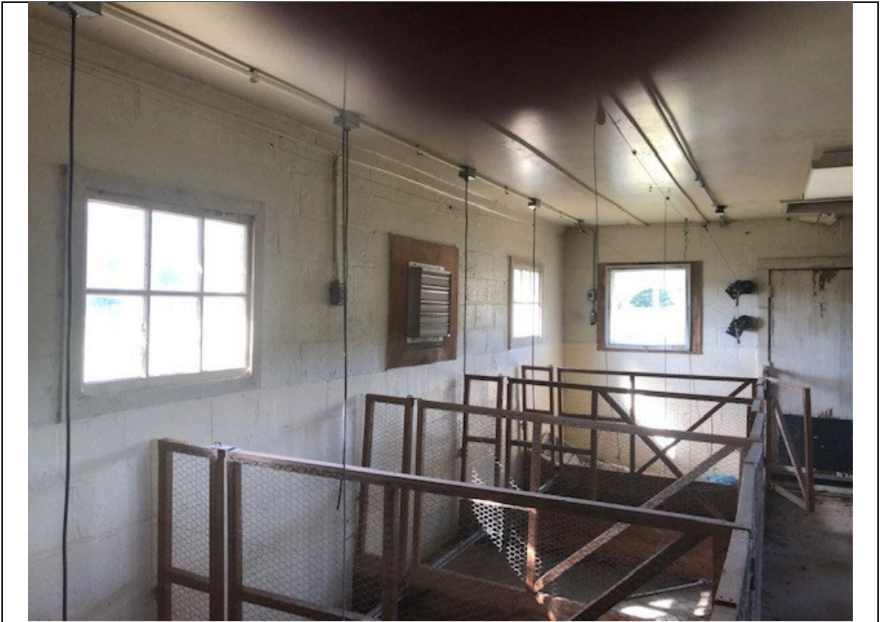
Interior – West End
