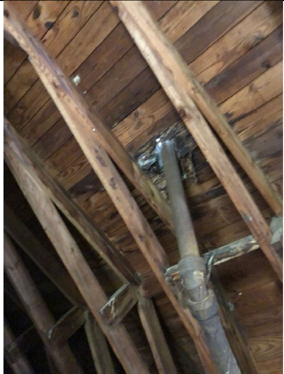
Attic – Damaged Wood Sheathing
