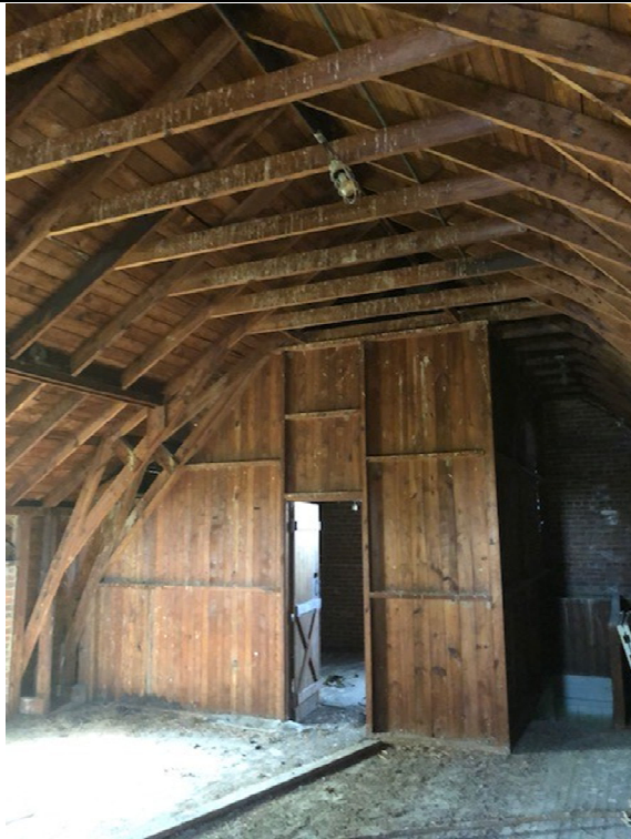
Attic – Looking West
