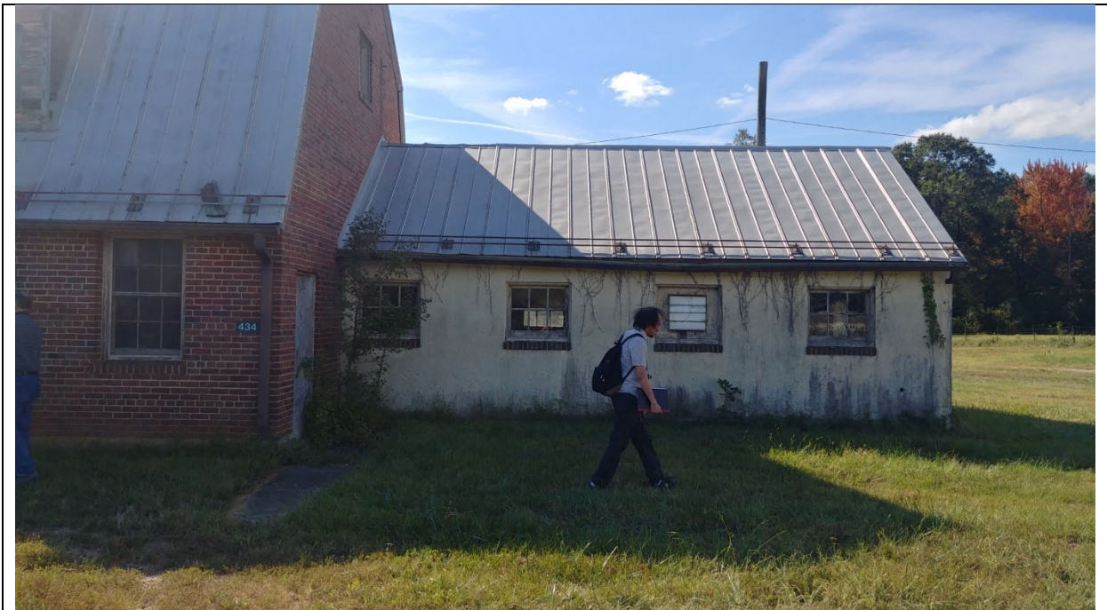
Exterior Elevation – North West End
