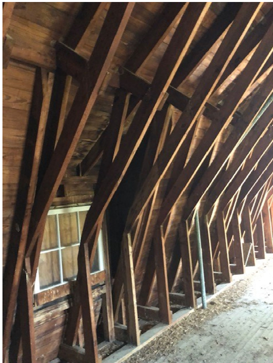
Attic – Dormers Over Wood Trusses
