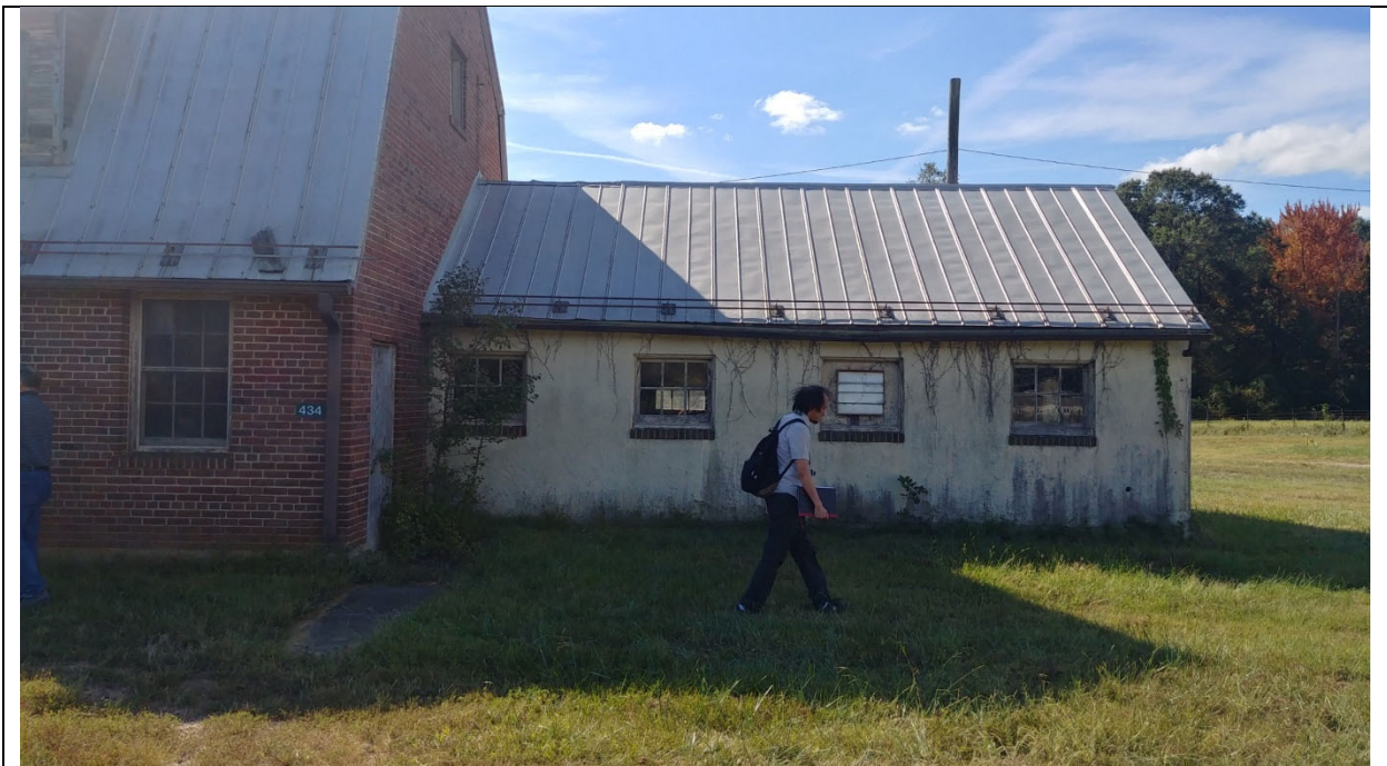
Exterior Elevation – North West End
