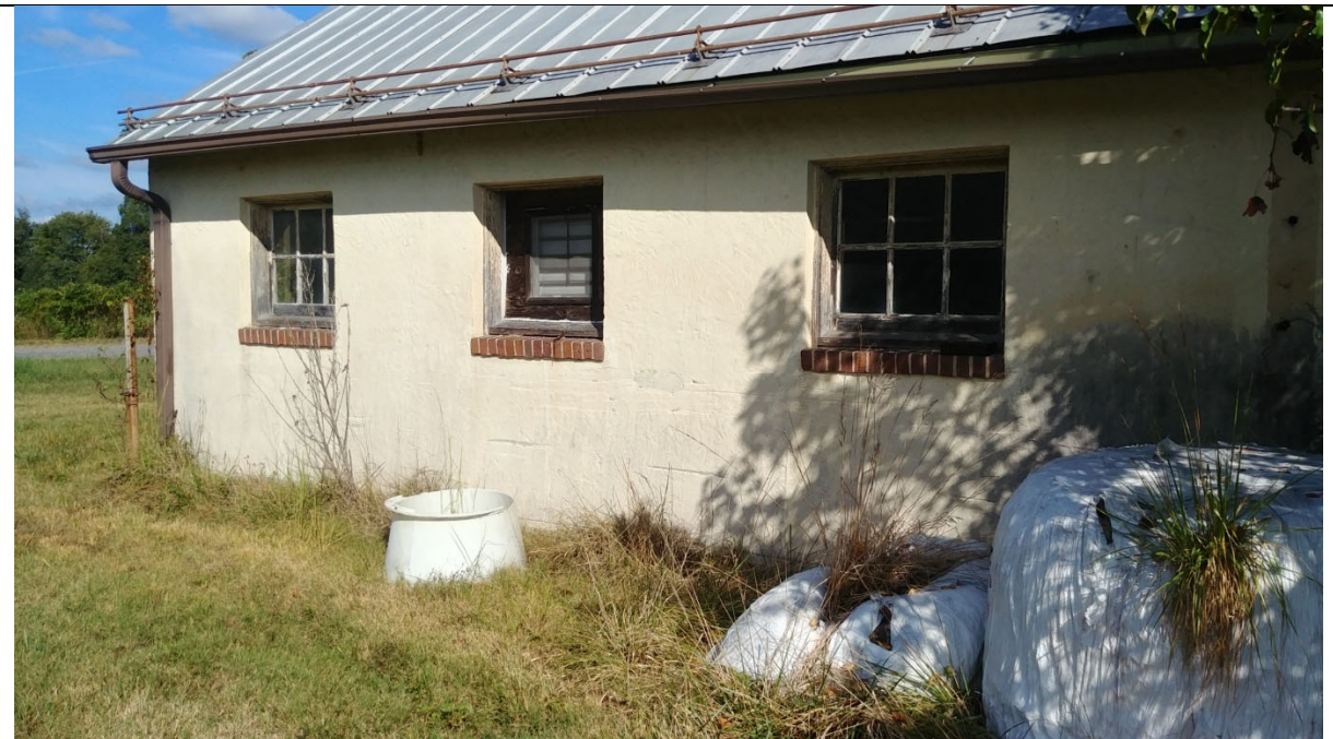
Exterior – South West End
