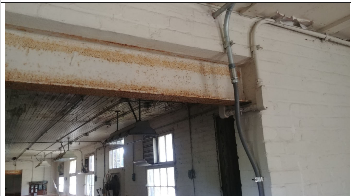
Original Interior Wall Was Removed
